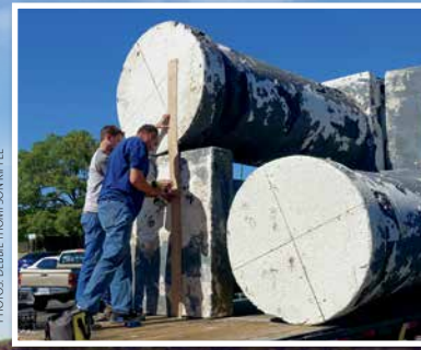
Using wood planks, the pillars were all tightly secured together.
